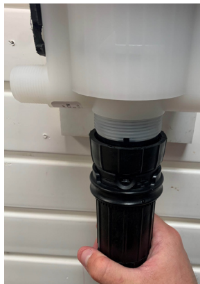
Step 8. Replace lower end assembly.
